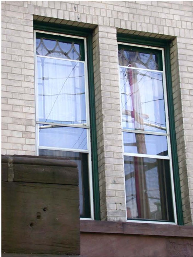
PLATE 13: Facade detail, front windows with upper sash with leaded glass.
