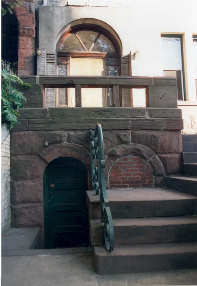
PLATE 15: Front entry, looking E.
