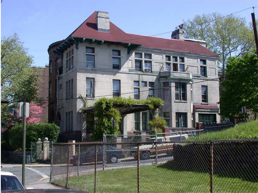
Plate 1: View of Green Gate looking NE.
