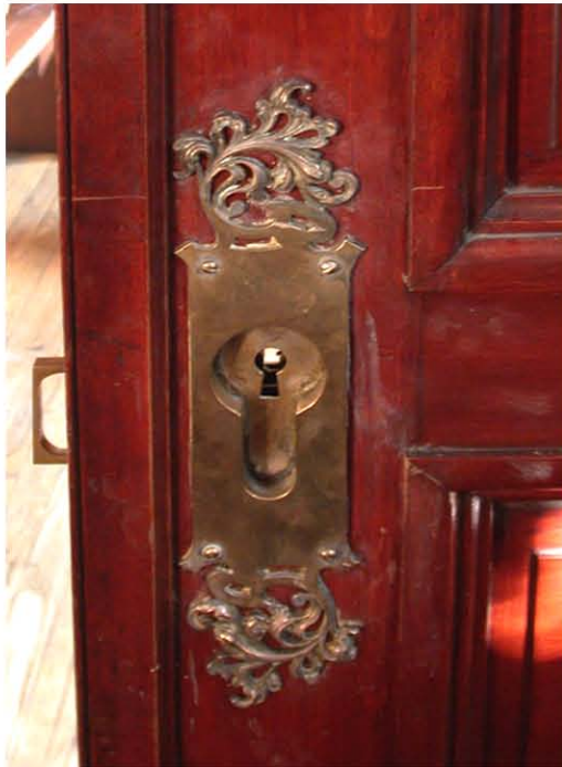
PLATE 41: Detail, ornamental escutcheon on pocket door, living room, looking E.
