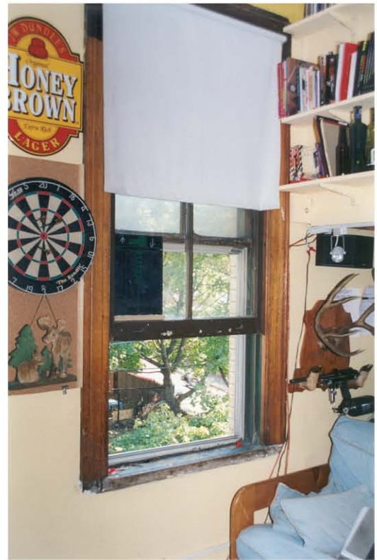
PLATE 36: Second floor bedroom at rear, looking SE.
