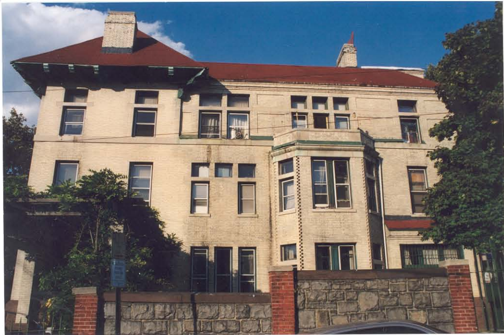
PLATE 7: South elevation with pergola and masonry wall, looking N from Eighth Street.
