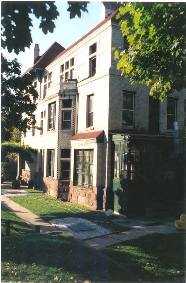
PLATE 3: View of south elevation and side yard, looking W.
