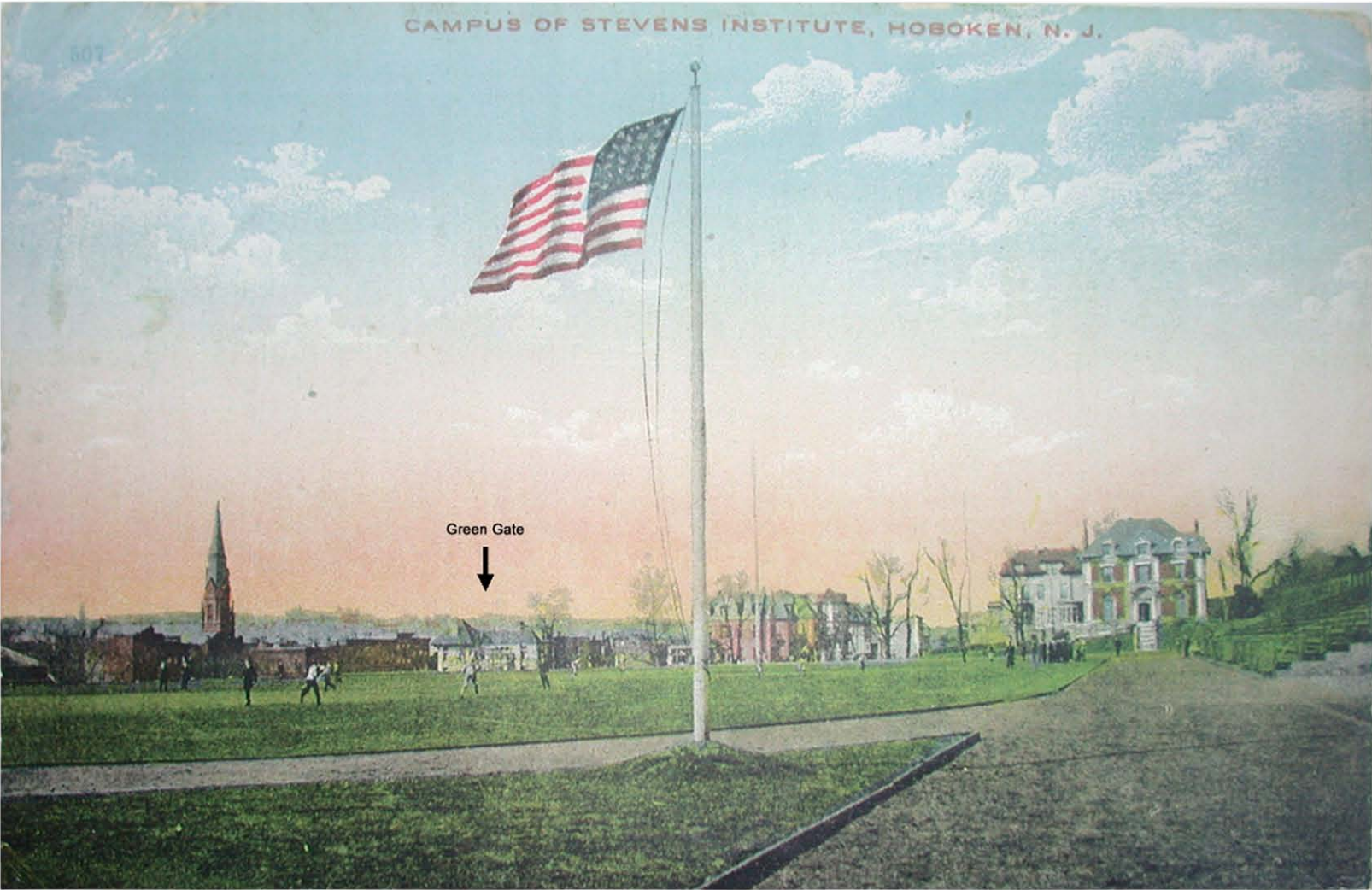
FIGURE 1: Historic postcard showing campus of Stevens Institute ca. 1910, showing Green Gate in background.
