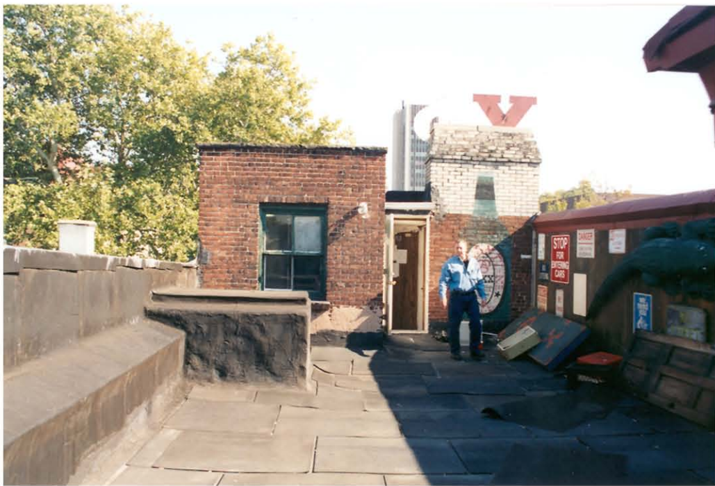
PLATE 44: Roof, looking E.
