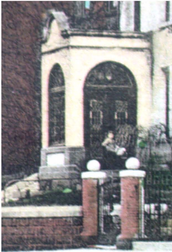
FIGURE 10: Detail front entry from postcard view circa 1912 showing leaded glass door panels and ornamental fanlight.
