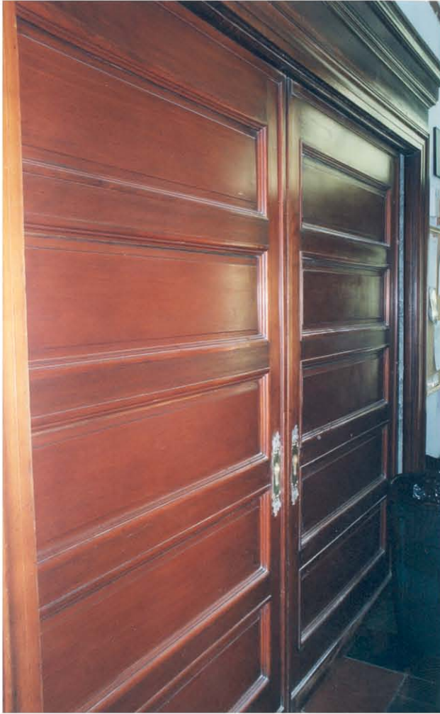
PLATE 23: Mahogany pocket doors between living room and front hall.
