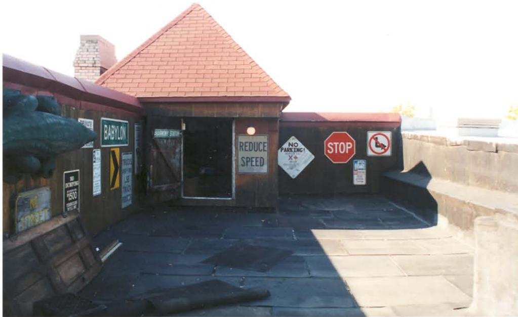
PLATE 43: Roof, looking W.
