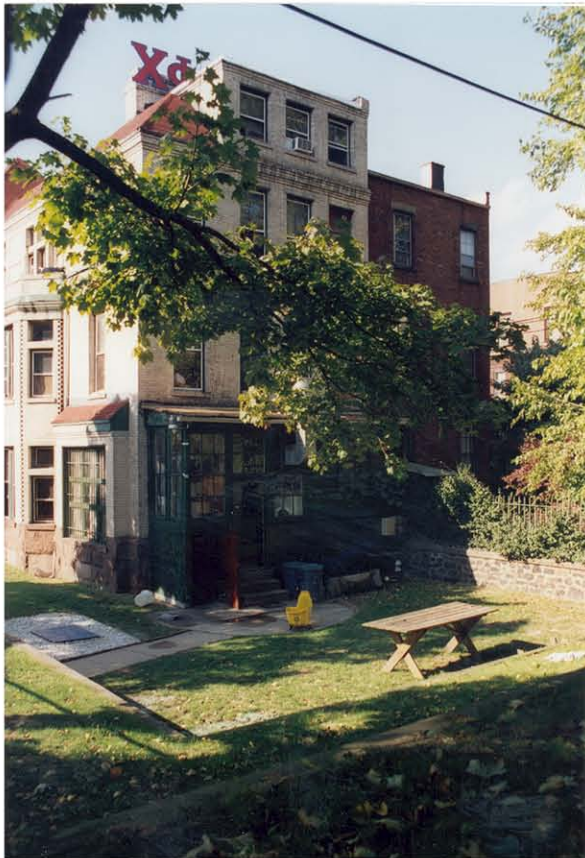
PLATE 18: Rear yard and east elevation, looking NW.
