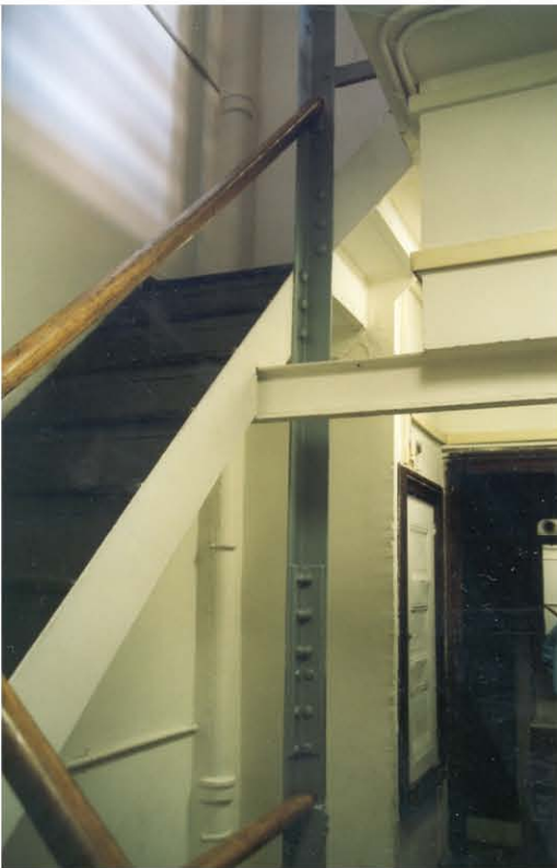
PLATE 33: Rear stairs between first and second floors, looking E.
