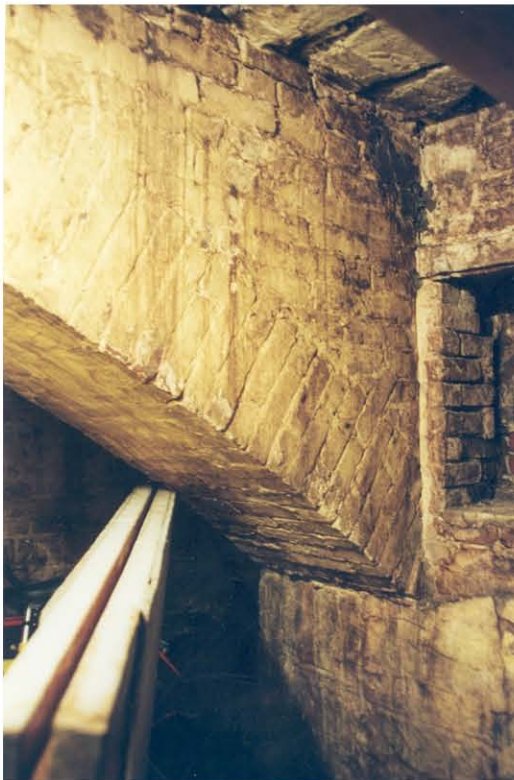
PLATE 37: Brick arch at front of cellar, looking SW.
