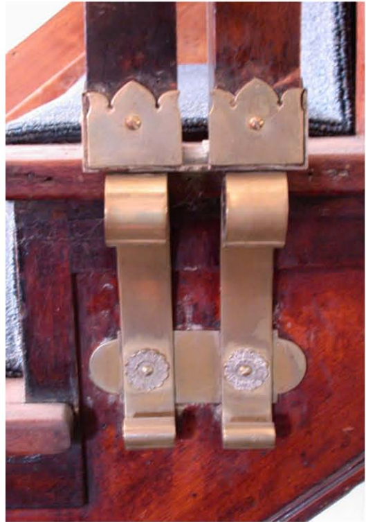
PLATE 40: Detail, brass baluster brackets on main staircase, looking N.
