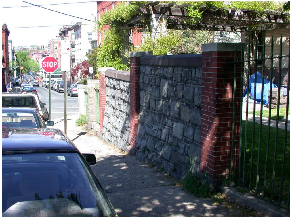
PLATE 8: Detail of two-bay masonry wall at former location of the Eighth Street stone gateway into the Stevens estate, looking W.
