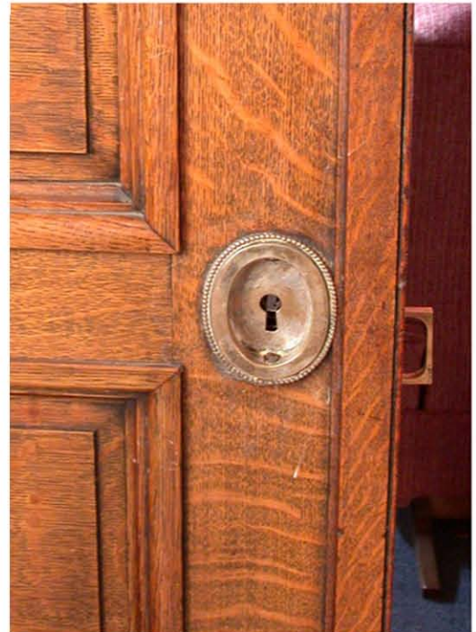
PLATE 42: Detail, ornamental escutcheon on pocket door of middle room, looking W.
