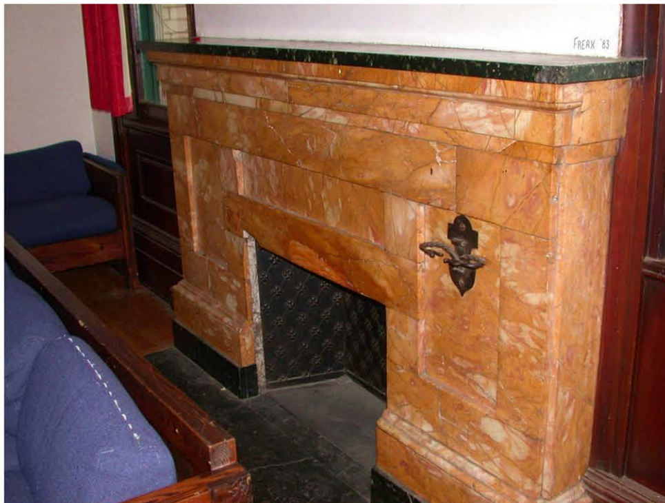
PLATE 22: Marble mantelpiece with wrought iron firetool tender and embossed cast iron lining, looking SE.
