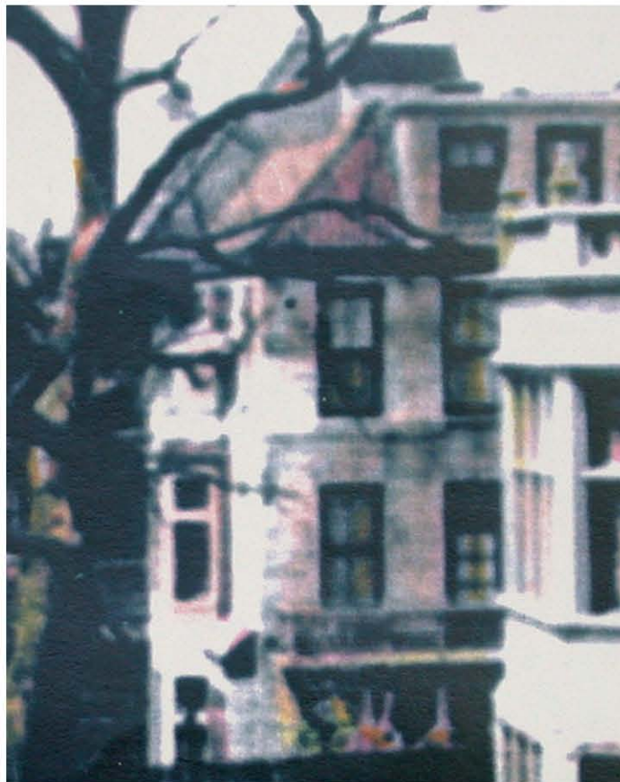
FIGURE 13: Detail of Fig. 12 showing 2/2 sash used in rear (east) windows of Green Gate.
