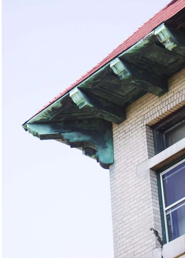
Plate 11: Facade detail: copper-clad modillioned cornice on corner pavilion looking NW.
