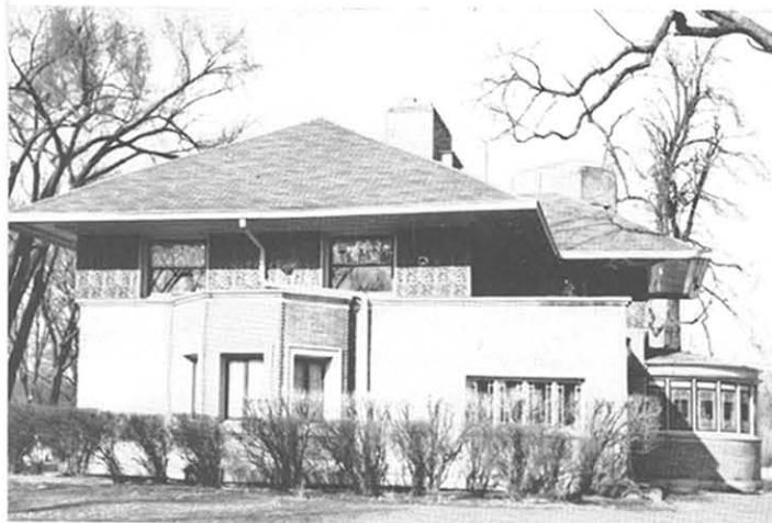
FIGURE 19: (At left) Side view, Winslow House, showing three-sided projecting bay.
