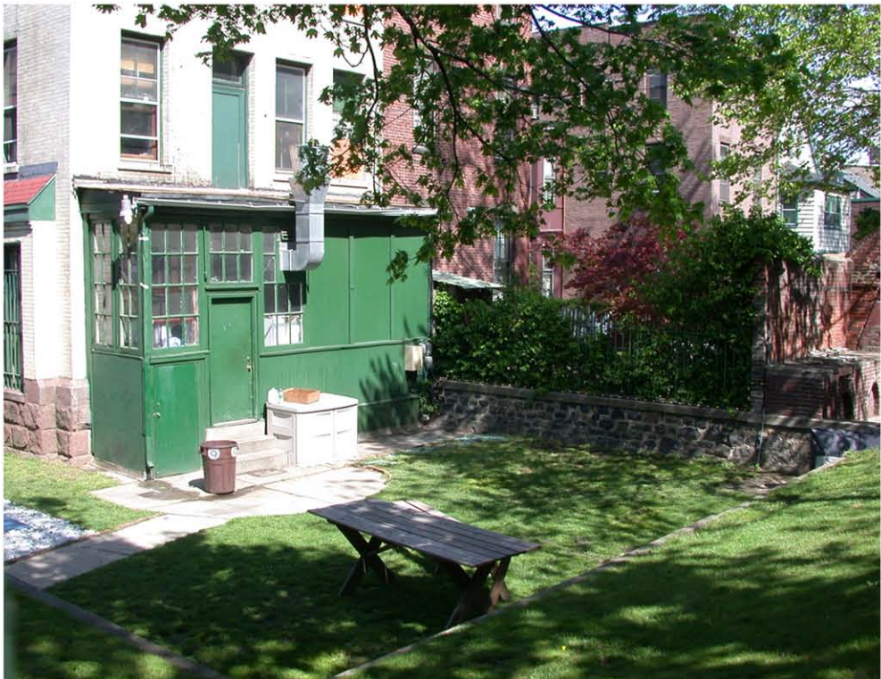
PLATE 4: Rear yard and porch, looking NW.
