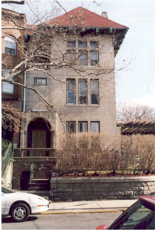
Plate 2: View of Hudson Street facade, looking E.
