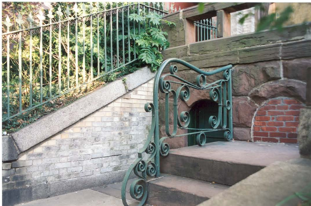
PLATE 16: Detail of wrought iron railing at Hudson Street entry, looking NE.
