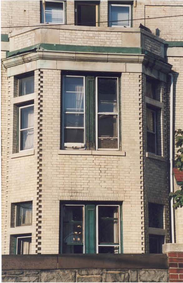
PLATE 17: Detail, three-sided projecting bay on south elevation, looking N.
