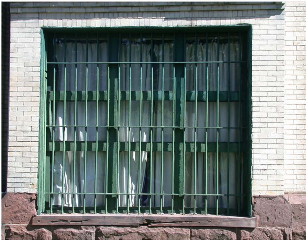
PLATE 14: Detail of south elevation showing windows in study room, the former conservatory,
