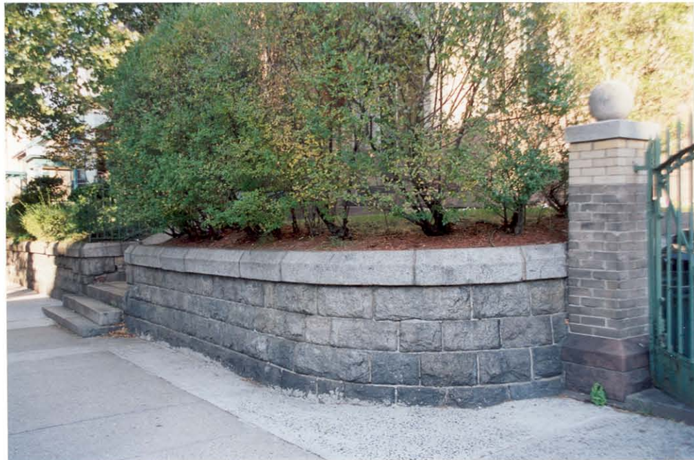
PLATE 6: Masonry retaining wall along Hudson Street, looking N.
